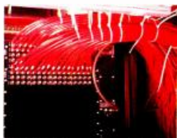
WLVI-TV has installed Mohawk/CDT Spectrum coax cable.
